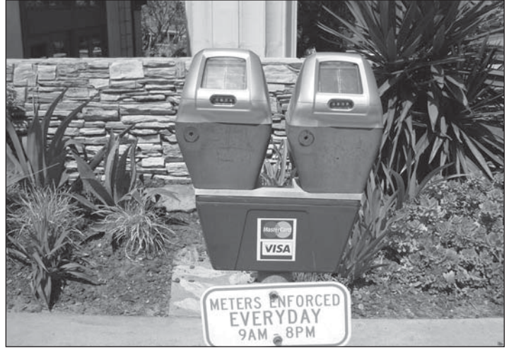
Solar Parking Meter. Photo Dan Nore
