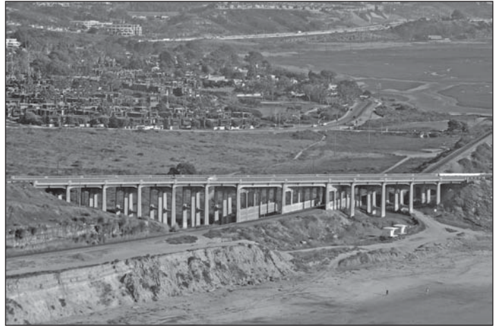
North Torrey Pines Bridge. Courtesy City of Del Mar.
